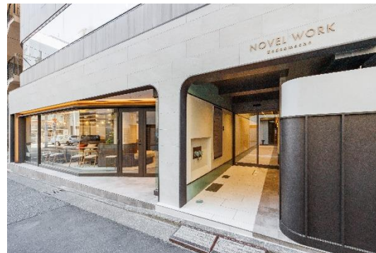
Renovated entrance with a sense of unity that matches the color tone of the office converted from the parking lot
