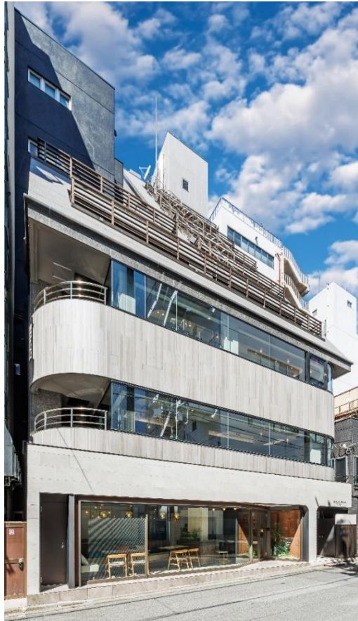
[Building exterior] Nihonbashi Kodenmachi, Chuo-ku, Tokyo 8-story steel structure building with deck roof
