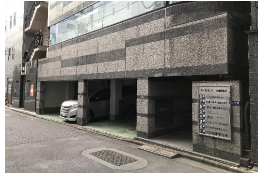
Parking lot on the first floor, which had been losing profitability due to low occupancy
