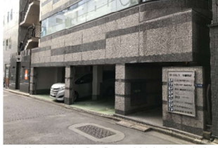
Parking lot on the first floor, which had been losing profitability due to low occupancy
