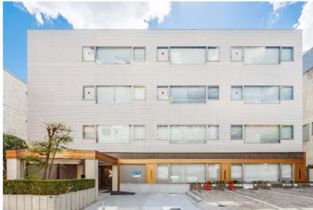
[Building exterior] Sendagaya Head Office Building, Shibuya-ku, Tokyo 4-story reinforced concrete building with deck roof
