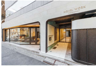
Renovated entrance with a sense of unity that matches the color tone of the office converted from the parking lot
